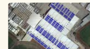
Installation of solar panels
