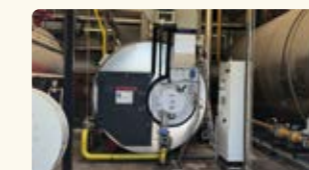
Installation of new-type boiler
